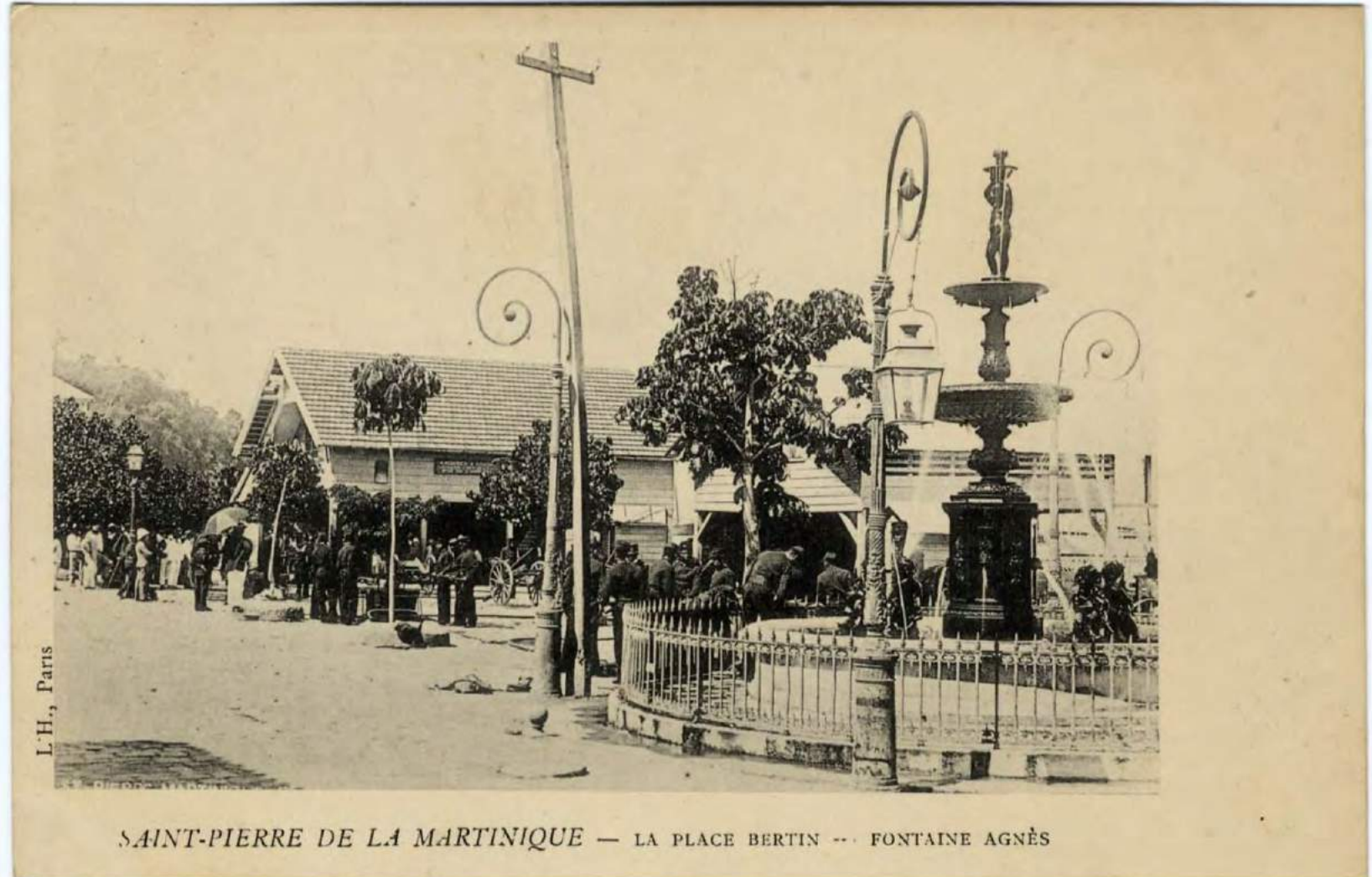
Water Fountain Agnès, Place Bertin on the waterfront (near the existing dock) – Note the electric street lamps
